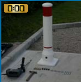
1) Position the bollard centrally on the intended site and orientate it correctly with regard to the site requirements.
