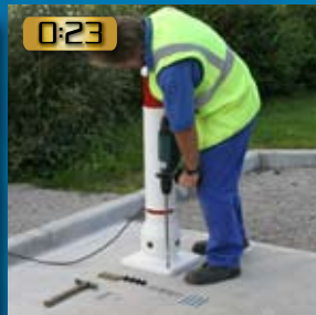
2) Using the bollard, mark out the four hole positions.
