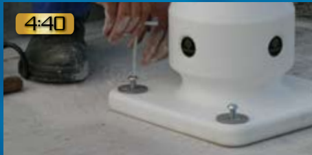
4) Insert the Anchor Rawl Plug, Spacer, Washer and Fixing Screw into each of the four holes. Using the 6mm Allen Key provided, loosely tighten each of the Fixing Screws.
